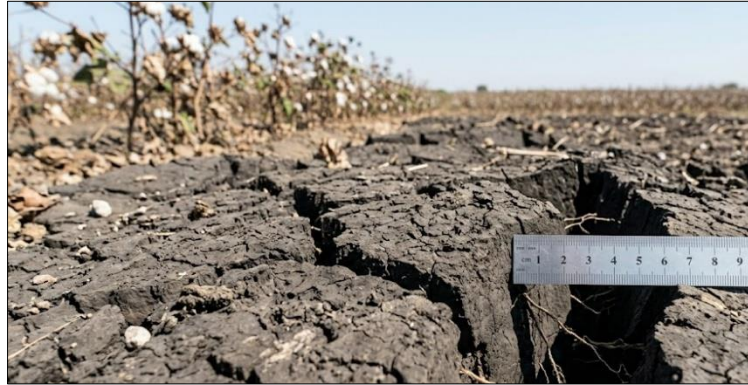
Fig 2: Close-up field photograph of hierarchical crack network in a Vertisol under cotton cultivation.
